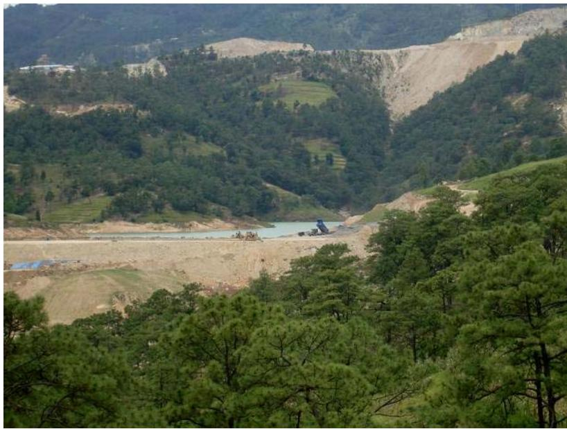
This photo shows the lake formed by the Marlin Mine, (the “tailings storage facility”), which is located in the lower part of the mine. The lake contains the process-affected waters which are now useless for the company. Clearly visible, the amount of water in the lake almost reaches the highest point of the dam.
